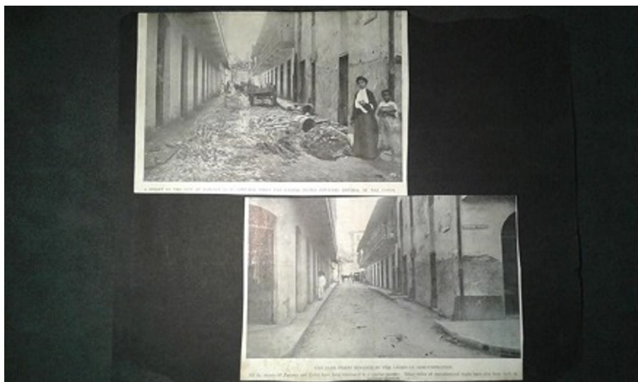
Fig. 6. Arriba: «A street in the city of Panama as it appeared when the United States obtained control of the canal.» Abajo: «The same street repaired by the American administration. All the streets of Panama and Colon have been renovated in a similar manner. Many miles of macadamized roads have also been built in outlying districts.» Image Archive, The Latin American Library, Tulane University.
