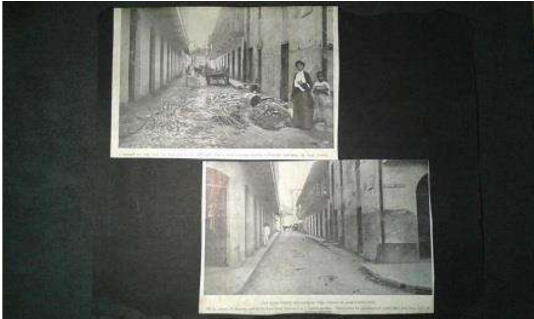
Fig. 6. Arriba: «A street in the city of Panama as it appeared when the United States obtained control of the canal.» Abajo: «The same street repaired by the American administration. All the streets of Panama and Colon have been renovated in a similar manner. Many miles of macadamized roads have also been built in outliving districts.» Image Archive, The Latin American Library, Tulane University.
